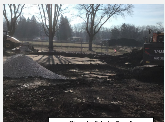
Sitework—Stripping Topsoil
