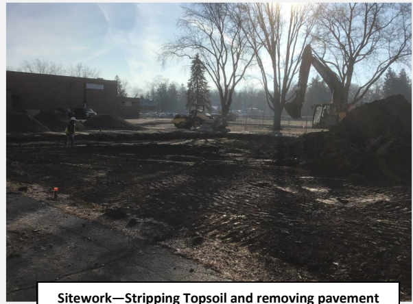
Sitework—Stripping Topsoil and removing pavement
