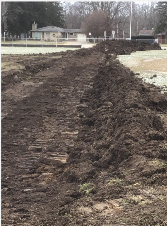
Sitework—Topsoil Stripped and Stock Pile
