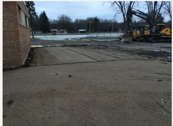
Site Fencing Around existing Trees
