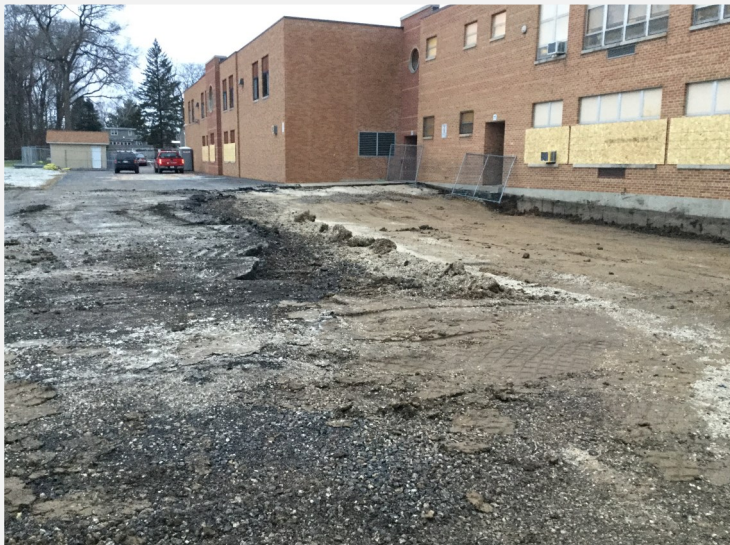
Sitework—Pavement stripped
