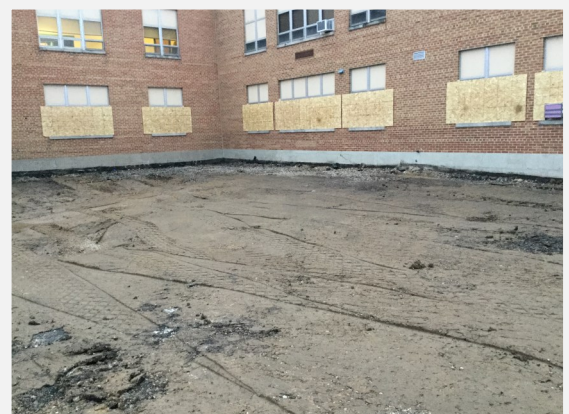
Plywood Protecting Windows
