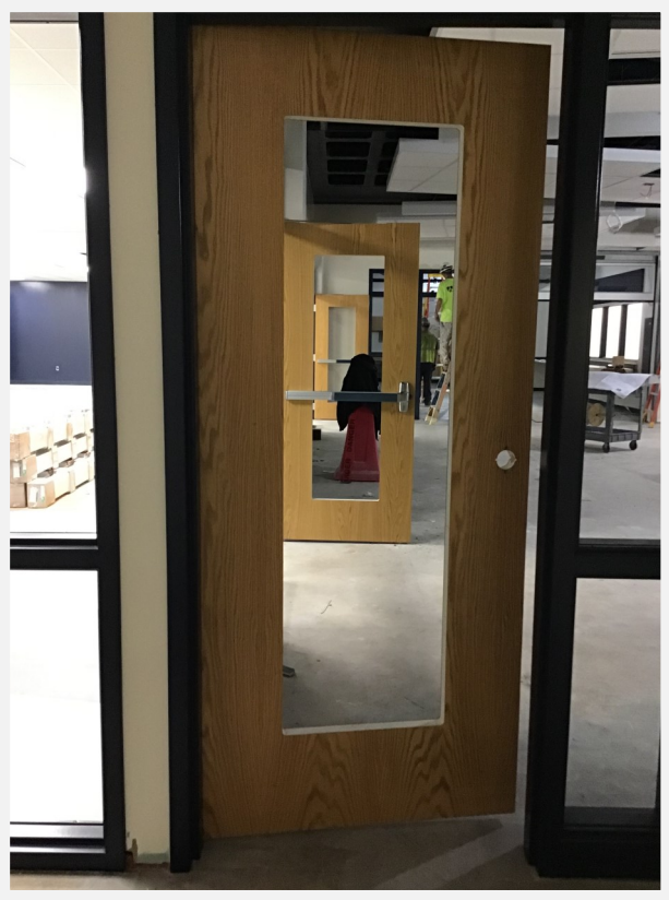
Doors and hardware are being installed.
