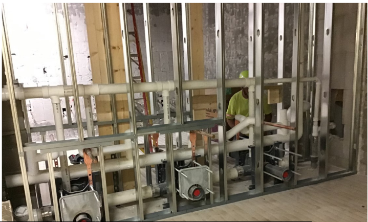
Toilet and Sink carriers installed and walls framed.
