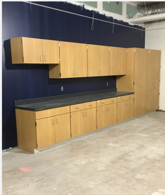
Looking into Science Classroom 113—Casework and ceiling grid is being installed
