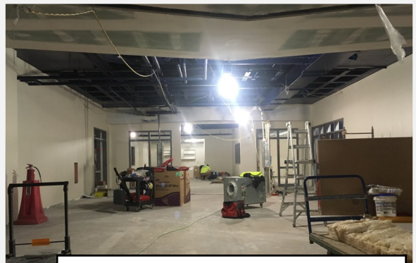
Looking into collaboration space—Walls mudded and taped and ceilings painted
