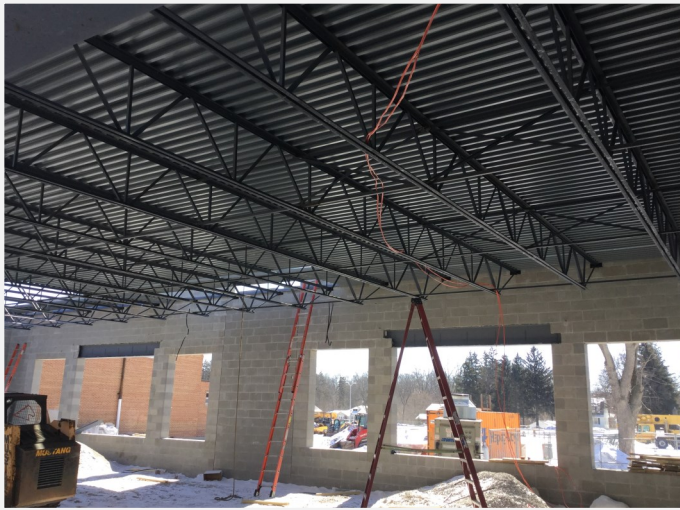
Steel Decking installed on top of joists (Picture of Kindergarten Room)
