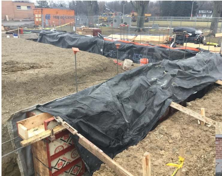
Foundation Wall formed, poured, and covered for frost protection
