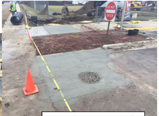
Storm Drainage System Connection
