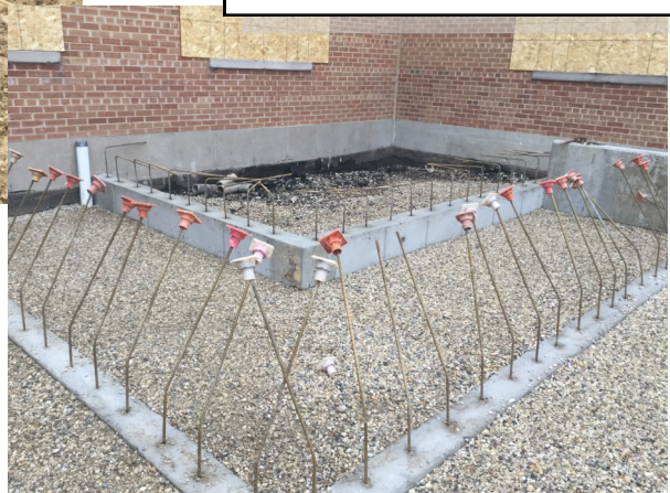
Courtyard Stair foundation walls backfilled
