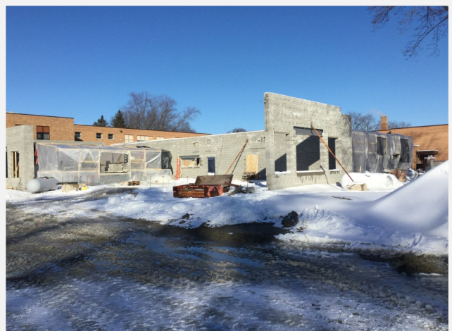
Overall Site Picture from South West Corner.
