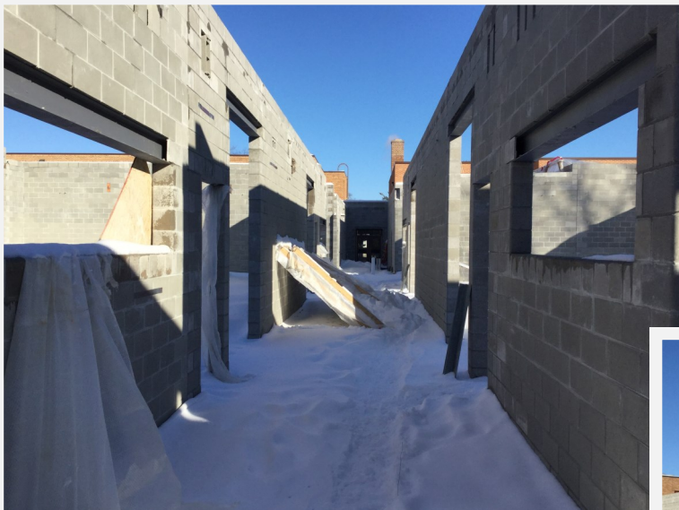
Masonry Block Walls— Corridor Running East/West
