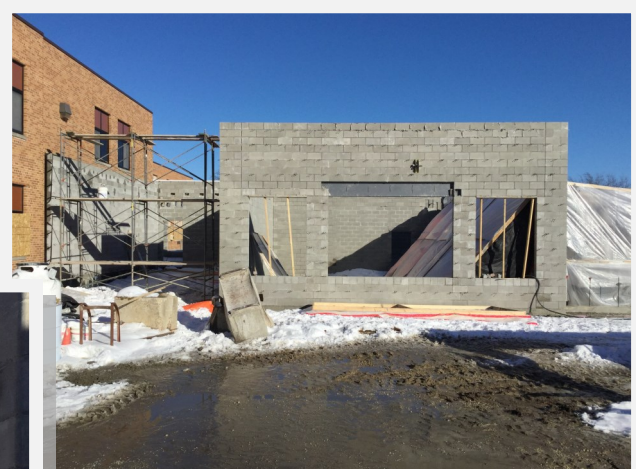
Masonry Block wall—Exterior Wall with Windows Looking west
