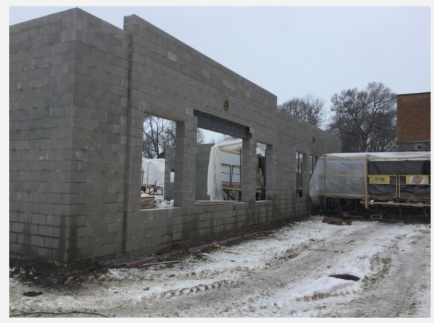
Masonry Block wall—Inside Courtyard—Looking South
