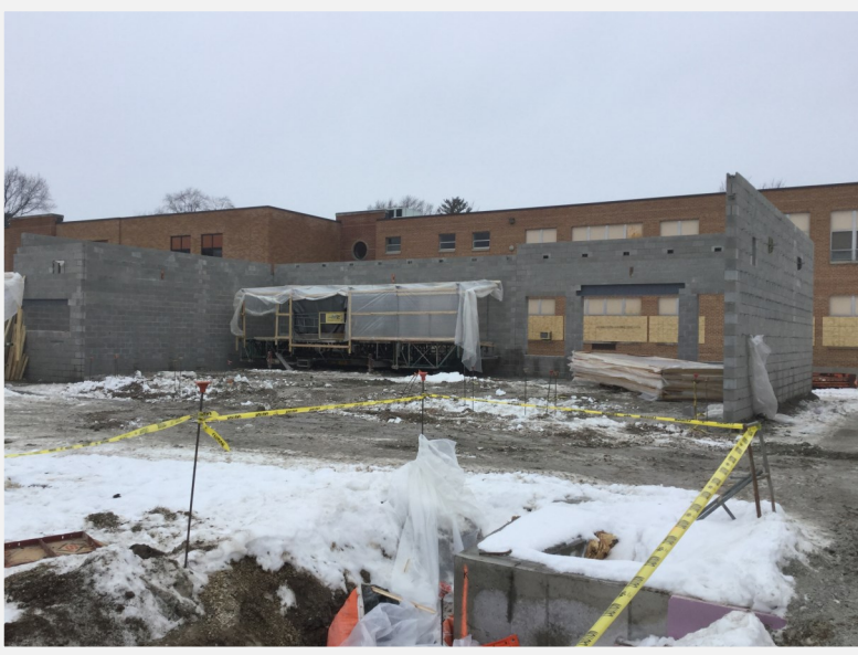
Masonry Block Walls—North Kindergarten Room
