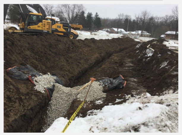
Temporary Storm Water Trench
