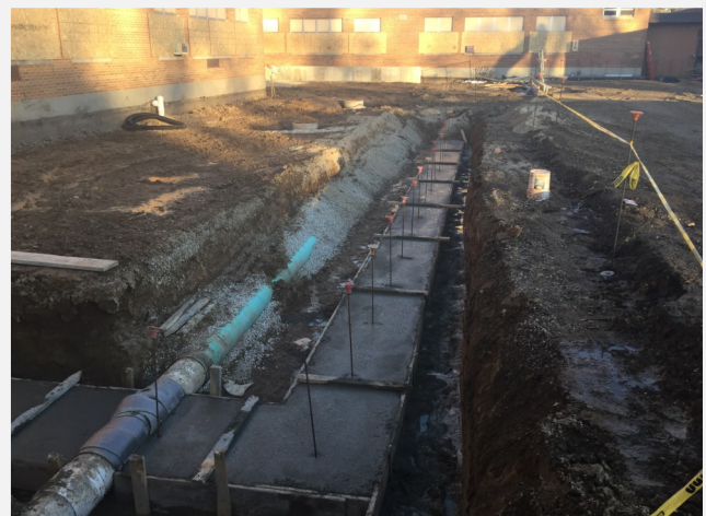
Classroom Footing Foundations
