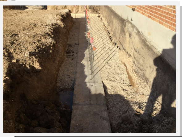
Footing forms stripped
