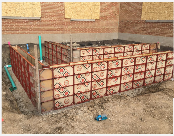
Foundation Wall Forms
