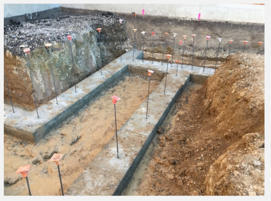
Courtyard Stair Footings Poured
