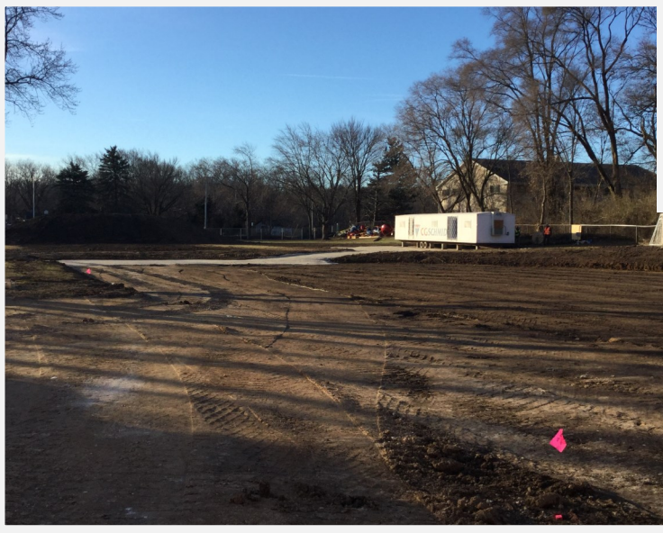
CG Schmidt Construction Trailer
