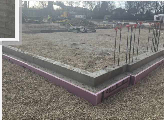
Footing/Foundation wall backfilled
