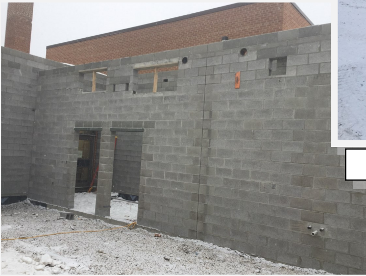
Completed Masonry wall, shows door openings and HVAC openings in wall
