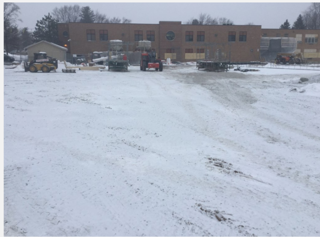
Stone Subgrade installed before major snow fall
