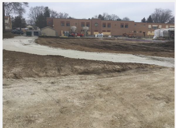
Access/Maintenance Road Subgrade
