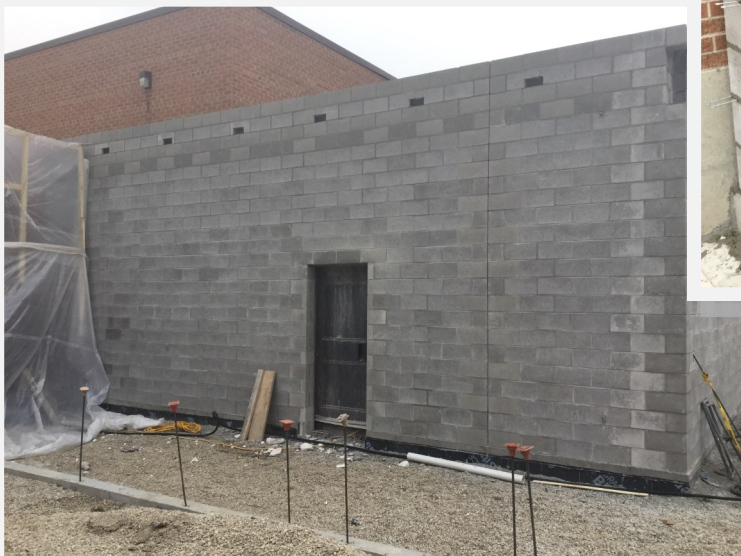
Example of completed Masonry wall
