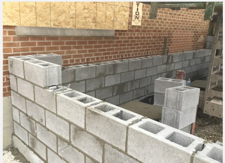
Masonry Walls being built.
